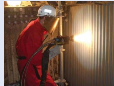
Protecting boiler tubes for the Power Generation Industry.
