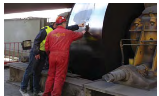
Extensive on-site wear analysis
