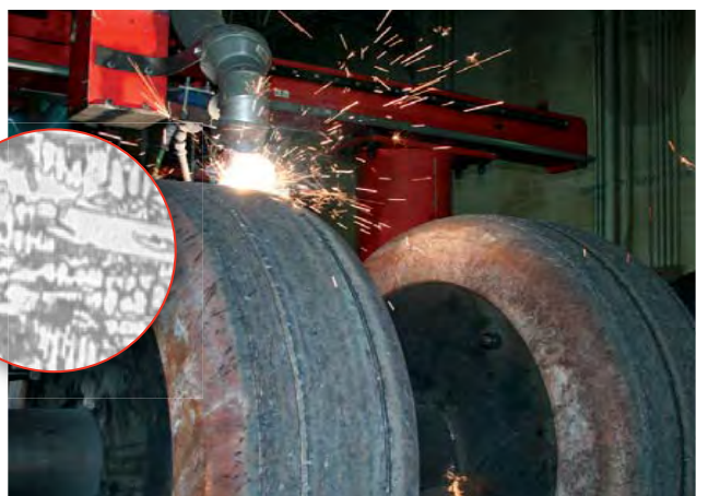
Automated Open-Arc Welding (TeroMatec®)
