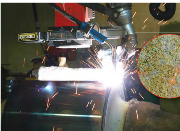
Automated Welding with Shielding Gas (EnDOtec®)
