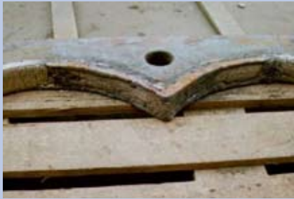
Worn areas on expansion center
