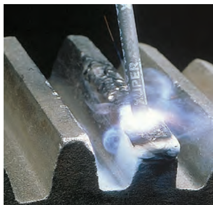
Casting defect repair
