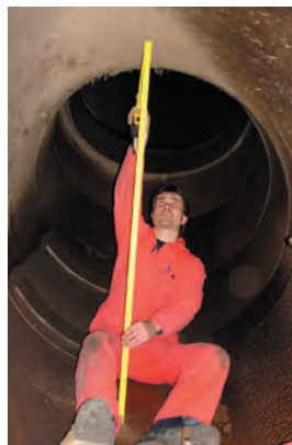
Repair in difficult conditions
