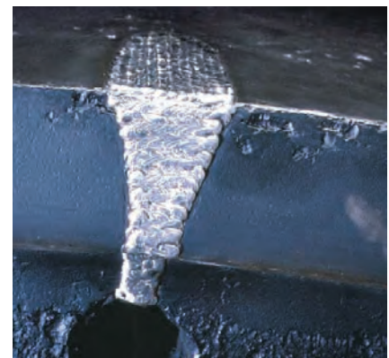
Low heat input and Xuper NucleoTec 2222 minimise residual stresses when performing massive repair welds on cracked cement kiln tyres.
