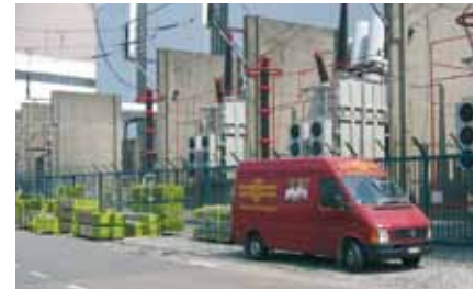
Local support at customer's plant
