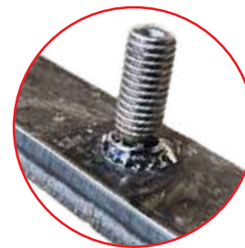
Welded Studs
