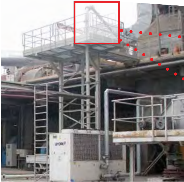
First line installation (passing through platform floor). Second line awaiting installation.
