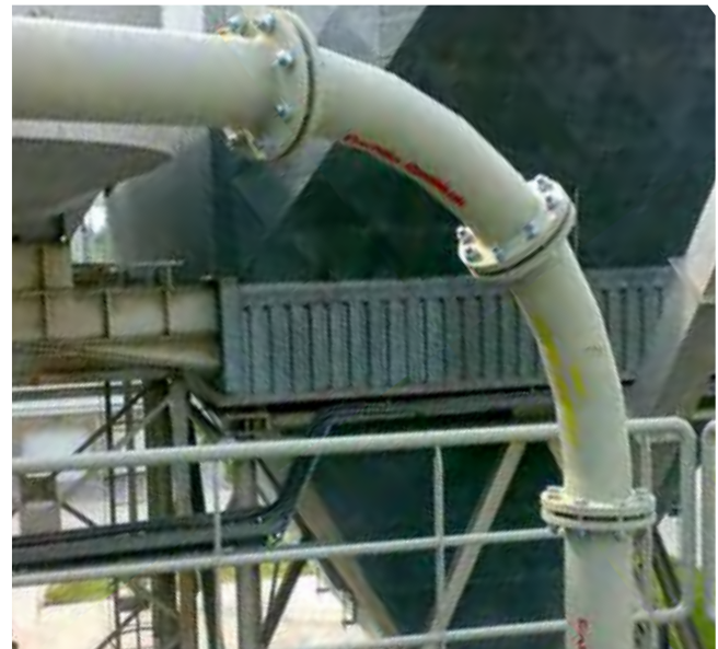
Elbows above the platform constructed from CastoTubes with NanoAlloy TM4395N coating have yellow inscriptions. Standard TM 4666 CastoTubes have red inscriptions.
