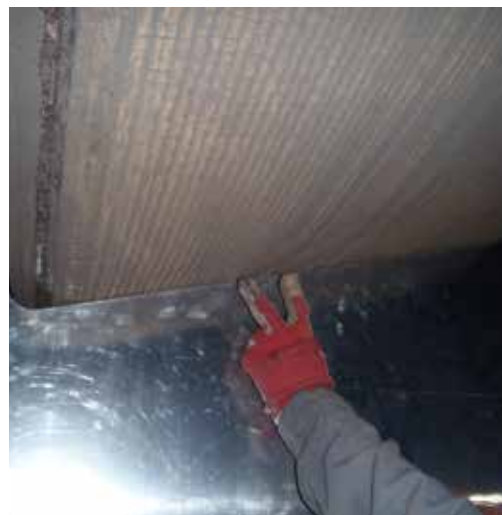
Checking the welded profile of a Loesche finishing mill
