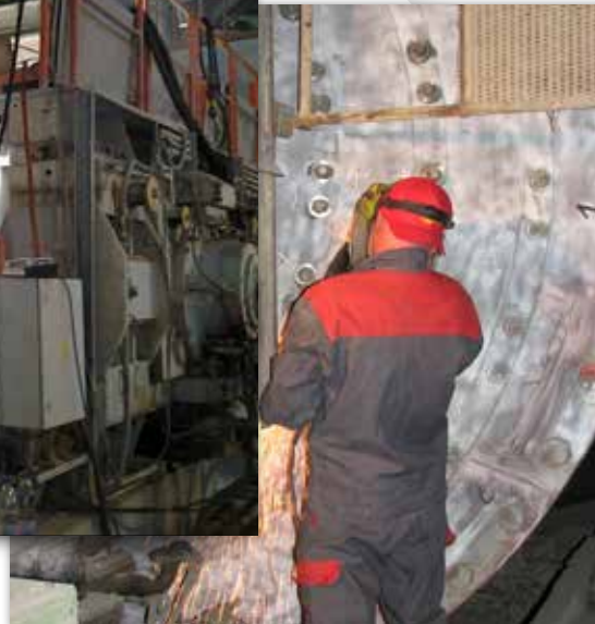
Crack repair of Ball Mill
