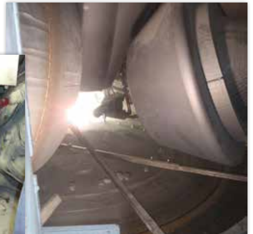
Loesche mill LM 46.2+2, 2 rolls and the table welded simultaneously
