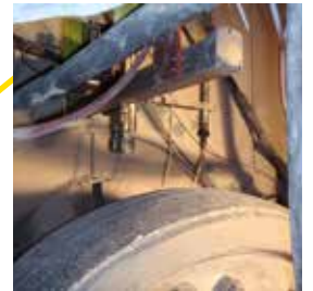
Repairing rollers with MTC 8338
