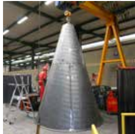
Coal mill cone repairs with CDP®
