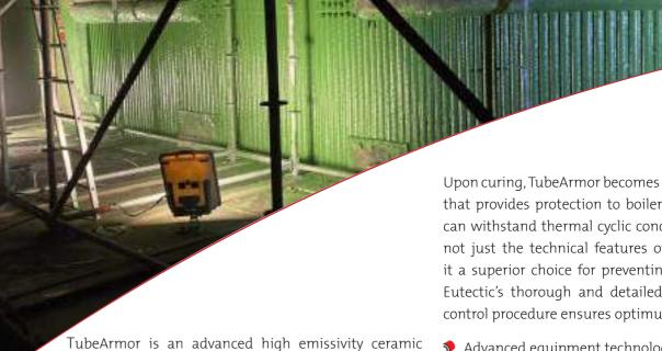
coating, specially formulated to provide erosion resistance and corrosion protection while increasing heat transfer and thermal efficiency. The coating is a high solids system which is applied as a stand-alone dry film at thicknesses up to 0.5 mm. It is thermally conductive and bonds extremely well to properly prepared steel substrates. TubeArmor is also applied over our ChromeClad thermal spray coatings.
